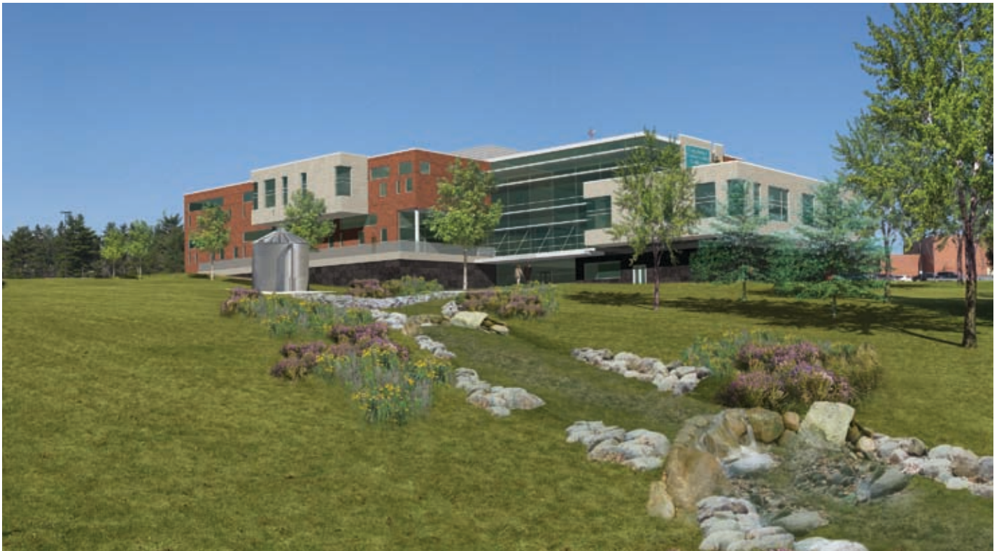
EASTERN CAMPUS HEALTH CAREERS TECHNOLOGY BUILDING: Cisterns, like the one above, provide a non-potable irrigation source. Vegetated swales slow water flow and reduce erosion to increase water quality as storm water moves away from the building above.
