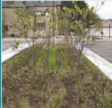
EXAMPLE OF A RAIN GARDEN located in a parking lot to detain and filter rainwater that flows from the parking lot.
