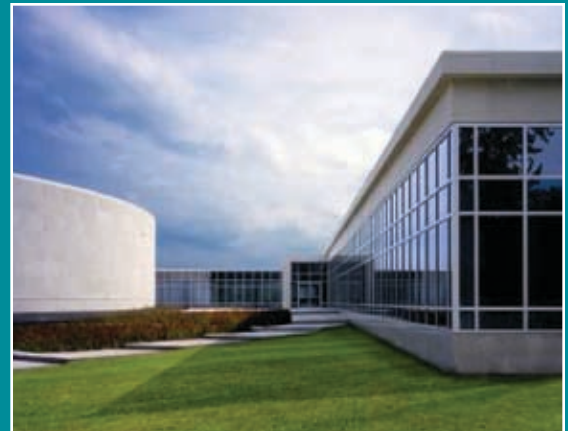
GREEN ROOF AT CORPORATE COLLEGE® EAST: Green roofs lessen the heat island effect, prolong the longevity of the roof and filter rainwater.
